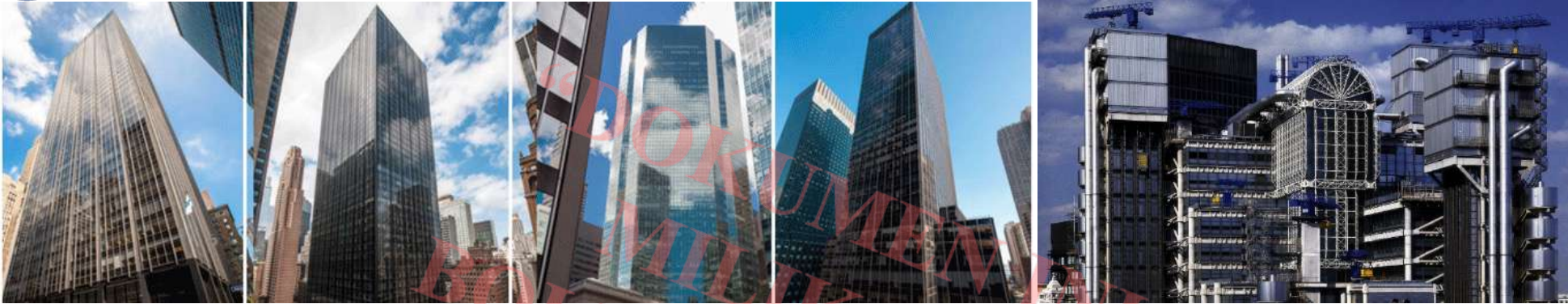
Four Fisher Brothers' Class A Office Buildings in New York ( link )
