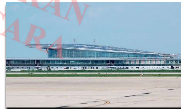
Hangzhou International Airport
